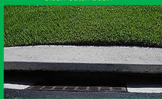
Clean Catch Basin
