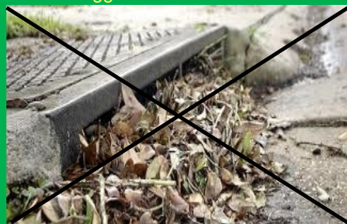
Clogged Catch Basin
